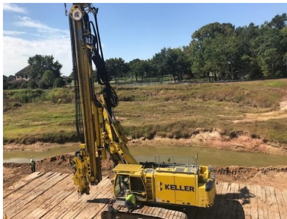
Phase 5- ABI Sheet pipe driver
