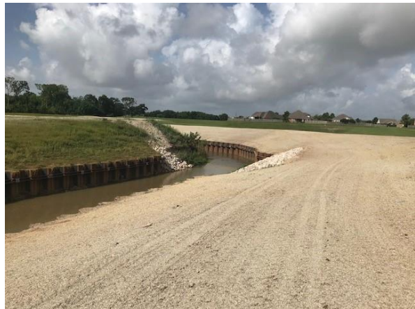
Phase 3 – Completed pre-vegetation
