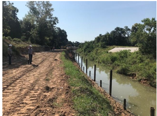
Phase 4 – Setting alignment piles for wall
