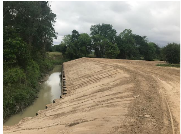
Phase 2 – Completed pre-vegetation
