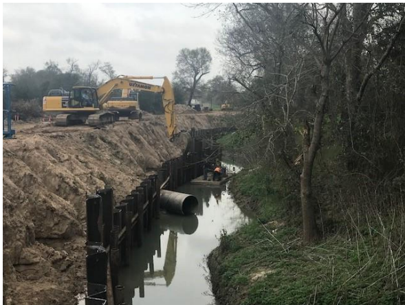
Phase 2- Waler installation
